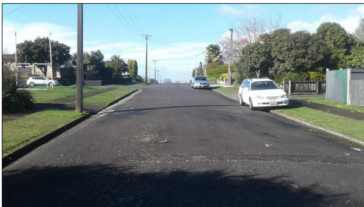
Figure 9: Cobham Drive / Stirling Drive Intersection Looking South
