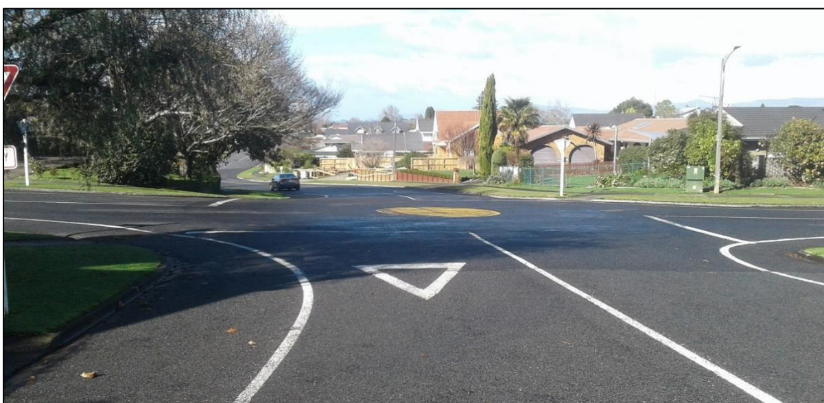
Figure 6: George Street / Stirling Drive Roundabout Looking South
