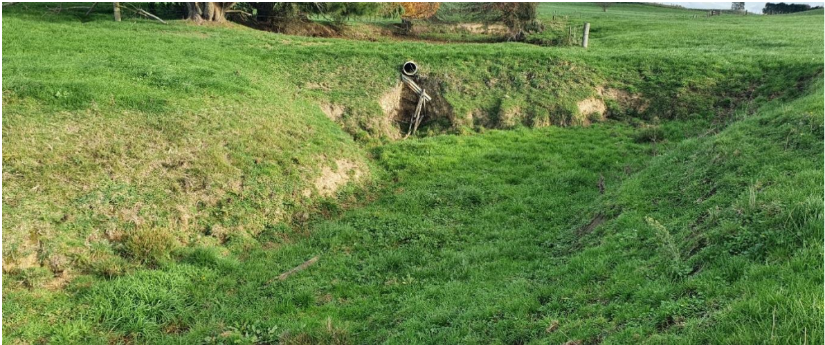
Figure 9: View of the upper section of Watercourse S3.
