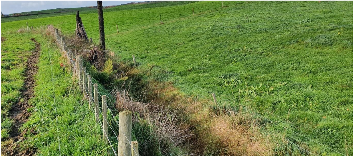
Figure 8: View of culvert 6 on Watercourse S3.
