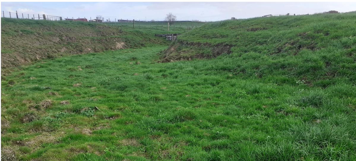
Figure 10: View of 'basin' upstream of culvert on Watercourse S3.
