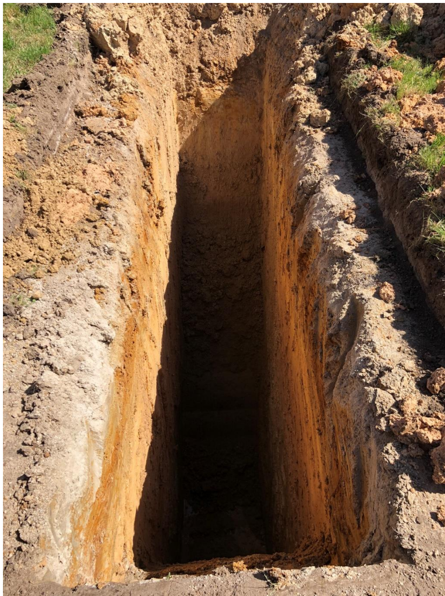
TP10 – TEST PIT EXCAVATION
