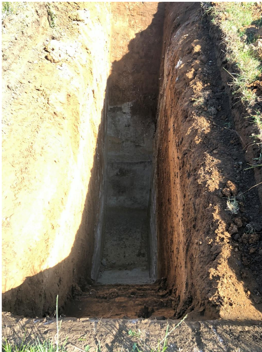
TP02 – TEST PIT EXCAVATION
