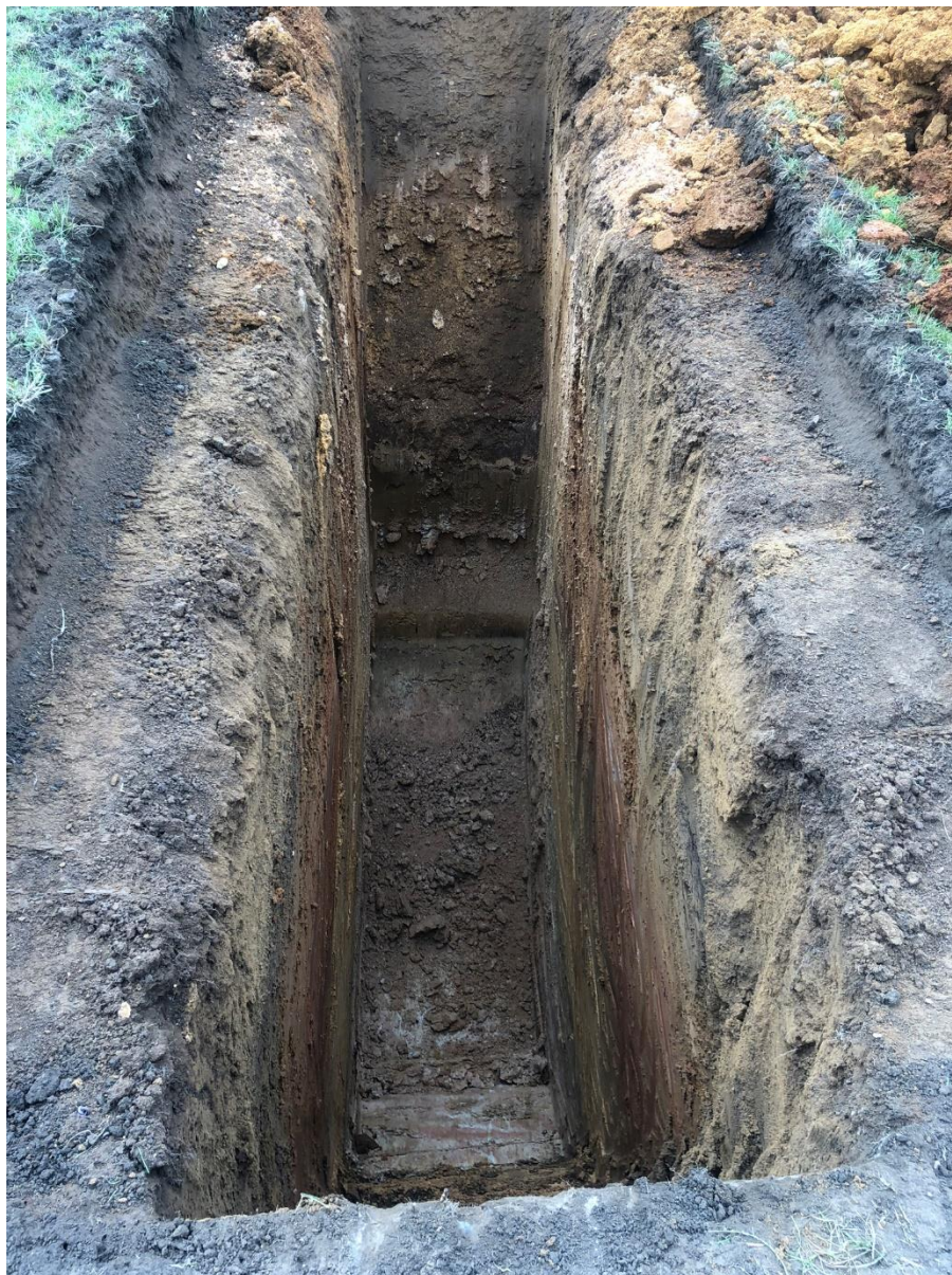
TP12 – TEST PIT EXCAVATION
