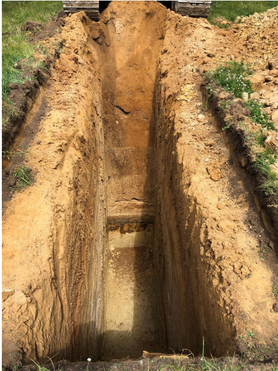
TP17 – TEST PIT EXCAVATION
