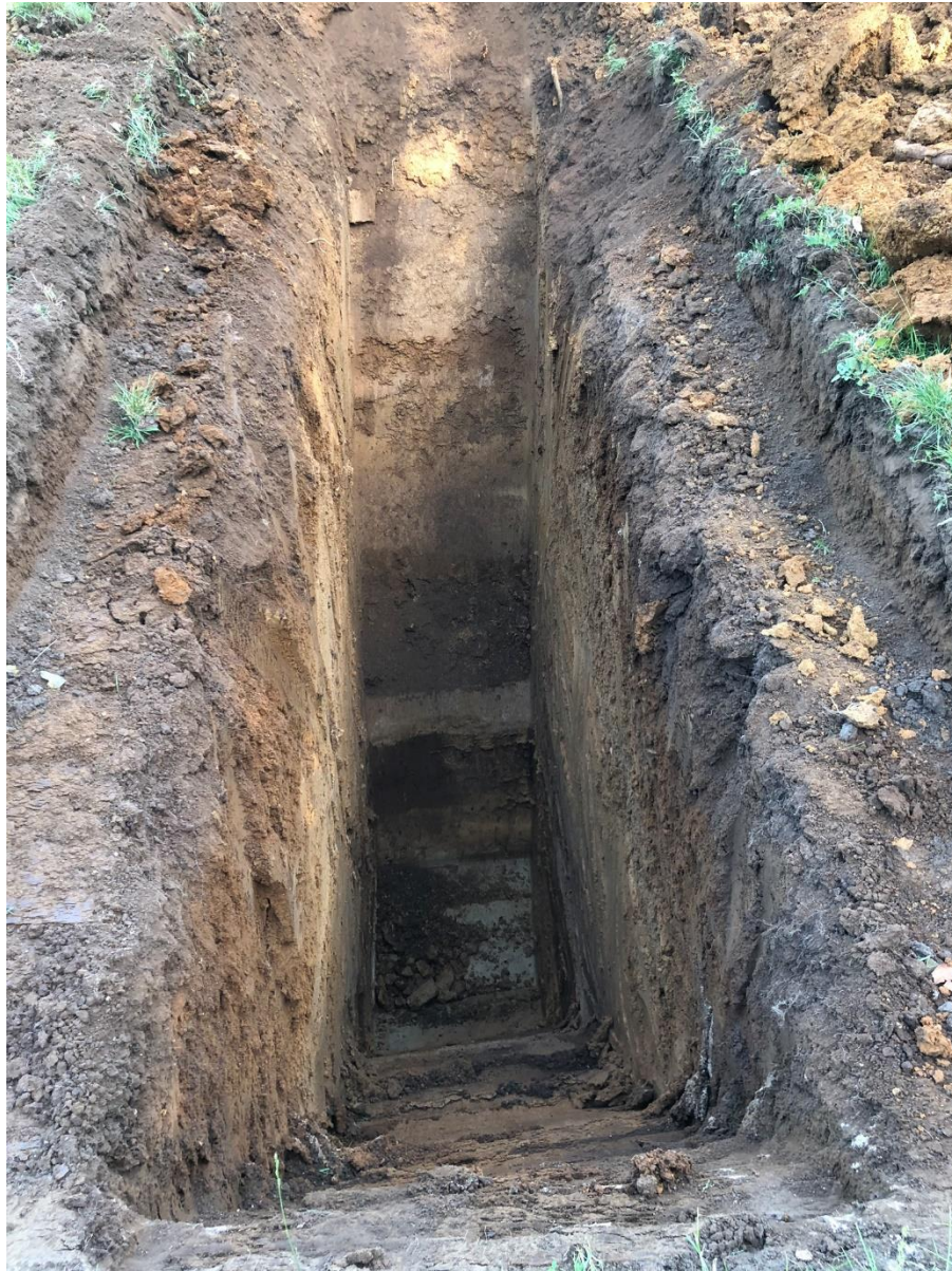
TP11 – TEST PIT EXCAVATION
