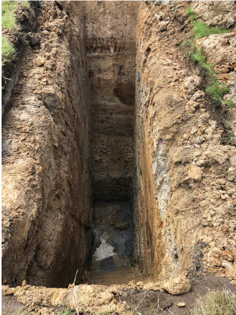
TP24 – TEST PIT EXCAVATION
