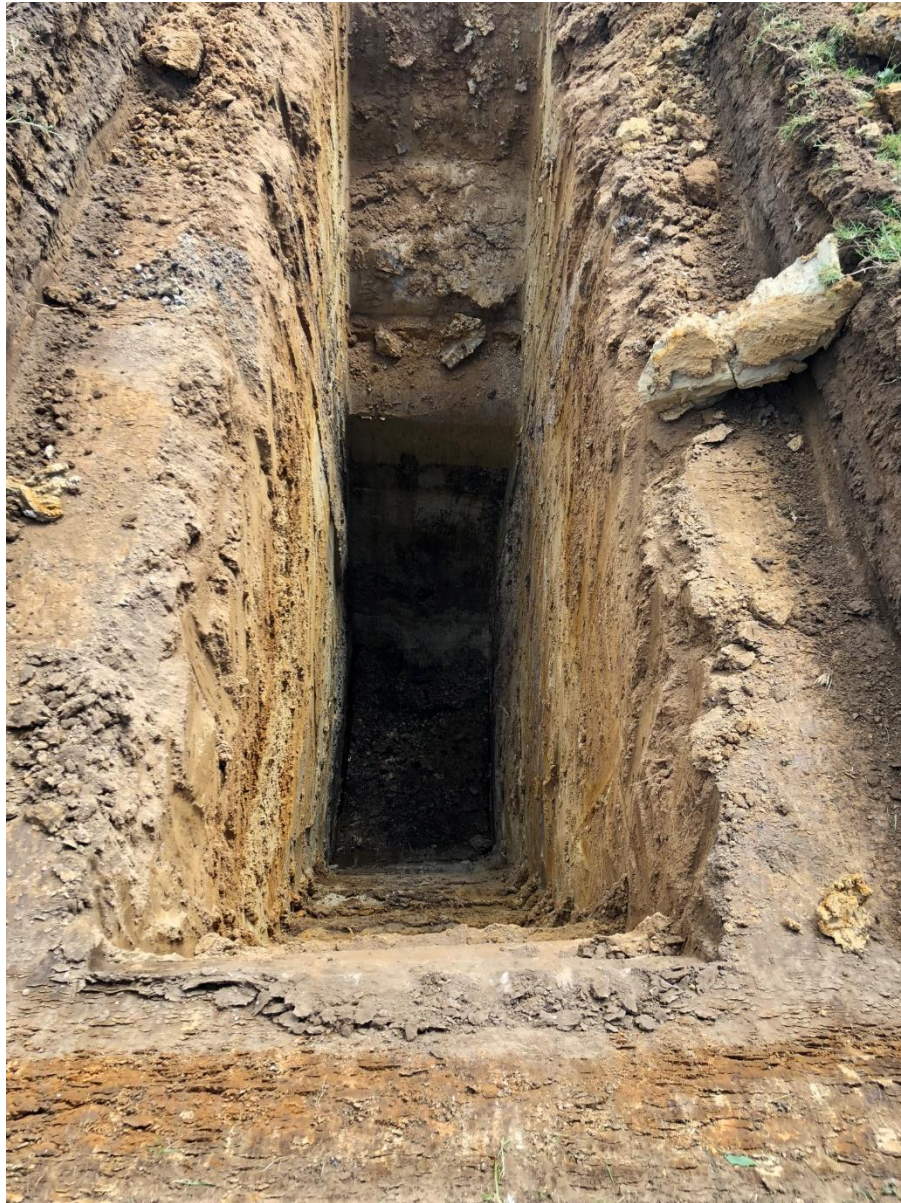
TP04 – TEST PIT EXCAVATION
