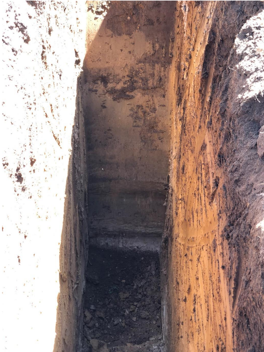
TP09 – TEST PIT EXCAVATION
