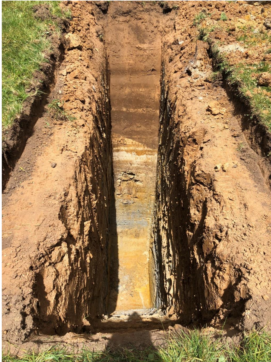
TP05 – TEST PIT EXCAVATION
