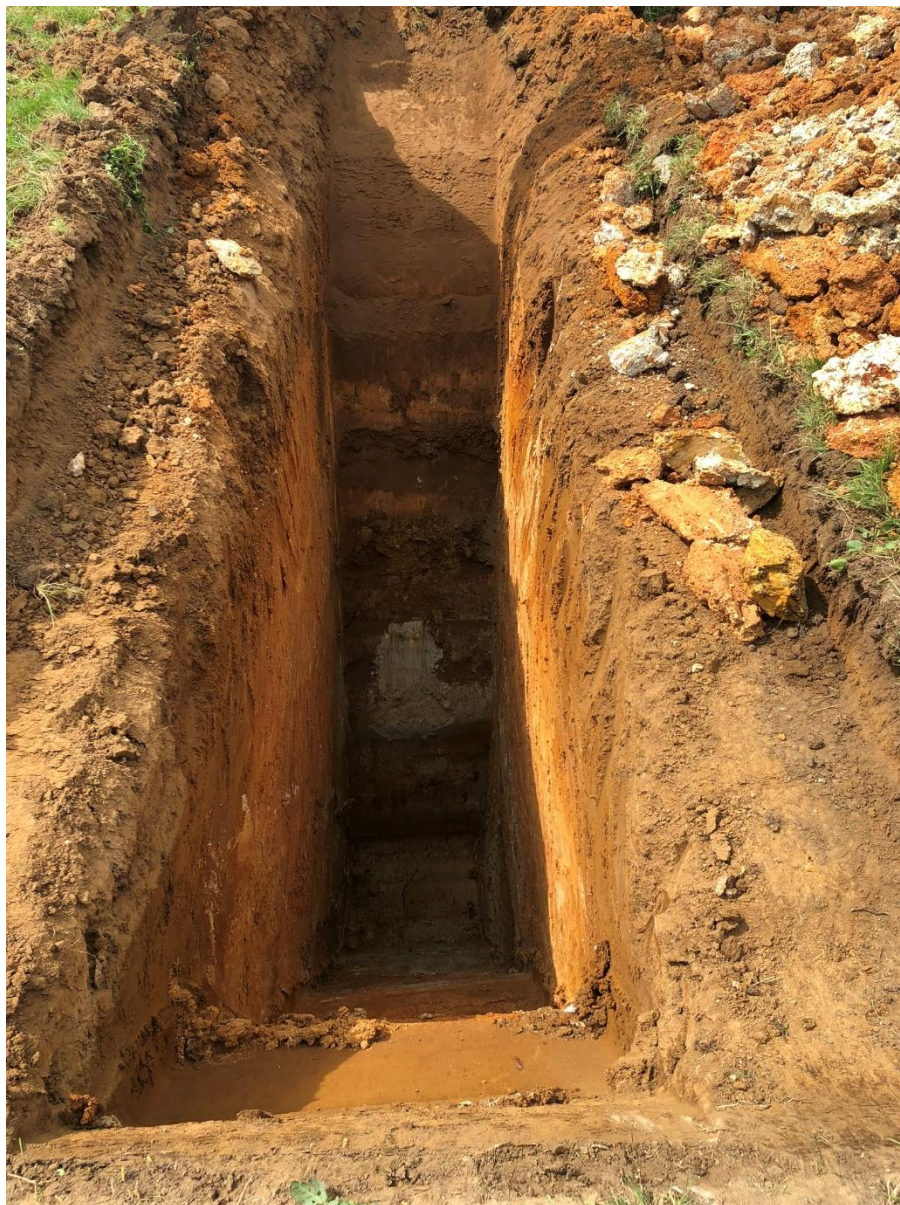
TP15 – TEST PIT EXCAVATION
