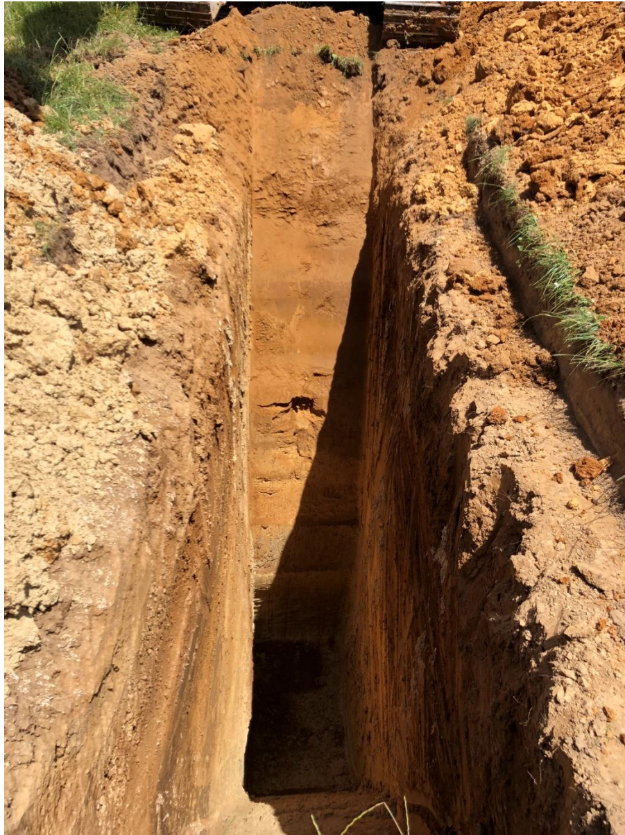
TP06 – TEST PIT EXCAVATION
