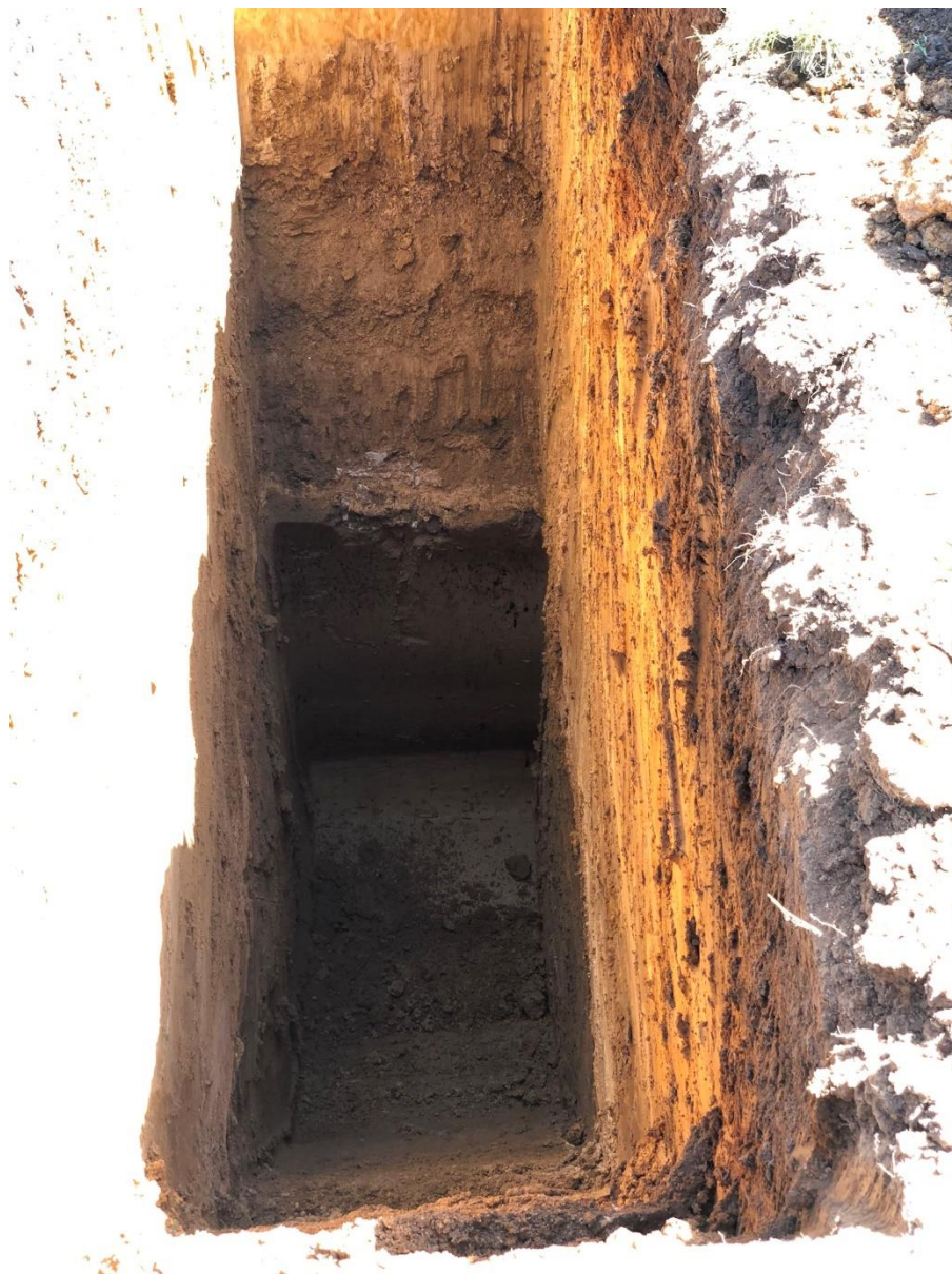
TP08 – TEST PIT EXCAVATION
