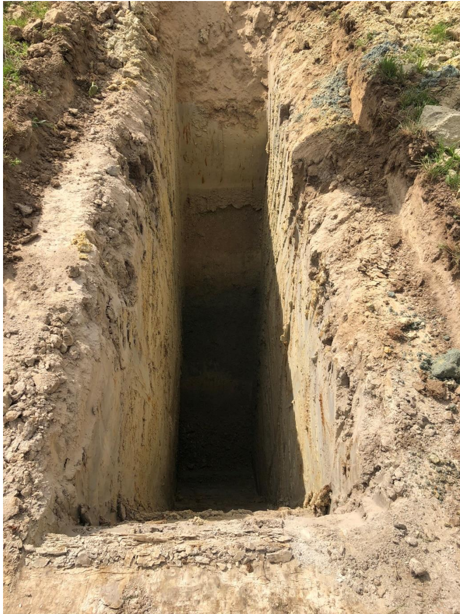
TP14 – TEST PIT EXCAVATION
