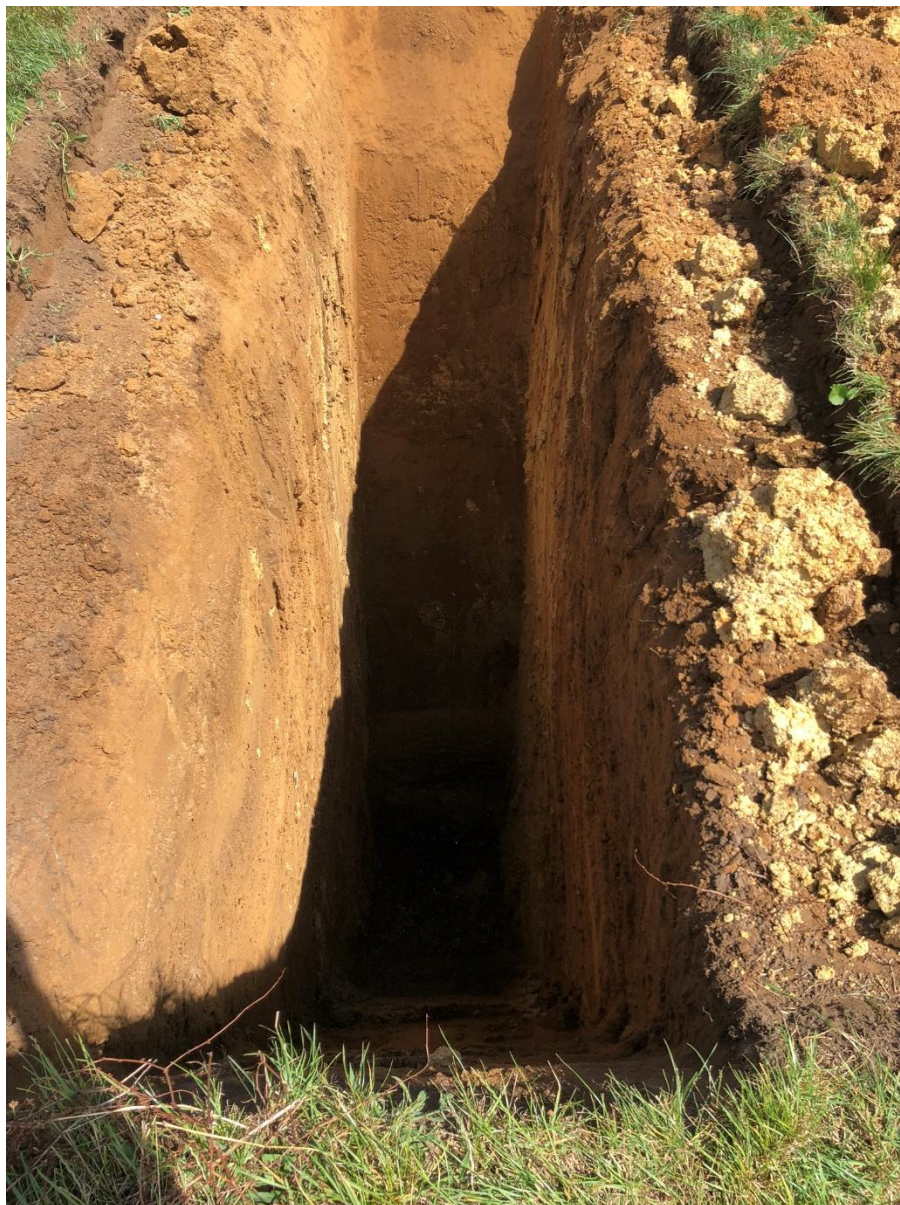
TP23 – TEST PIT EXCAVATION
