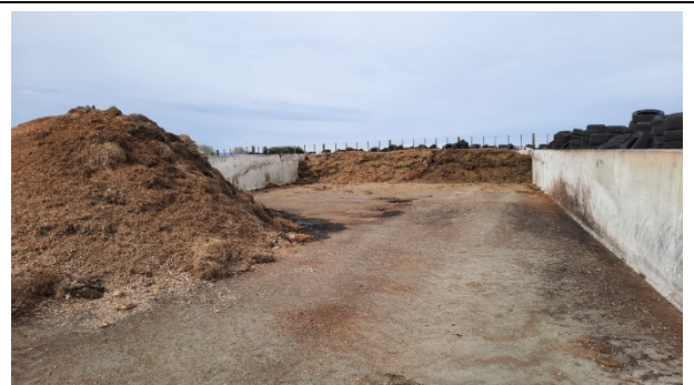
Photo 14: Concrete Feed Storage Area
