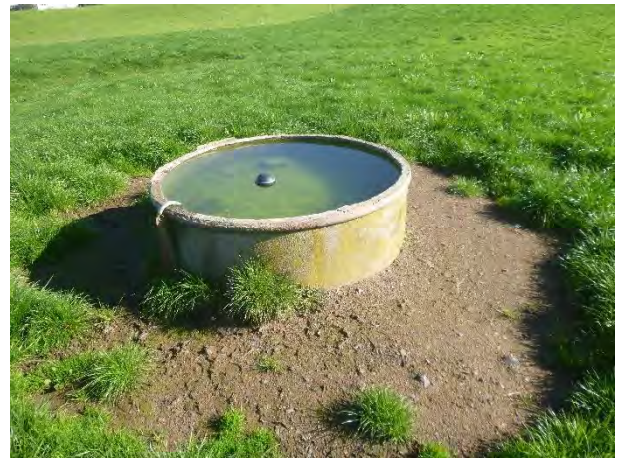
Photo 38: Typical concrete trough.
