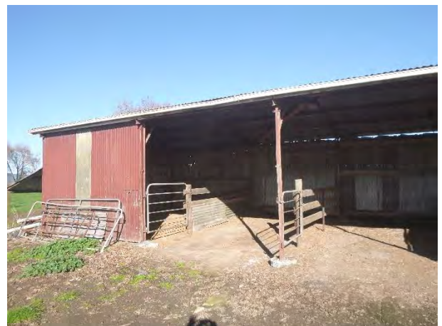
Photo 14: Metal farm shed.
