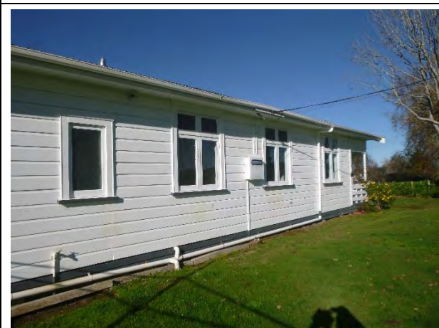
Photo 5: Northern side of the residential dwelling.
