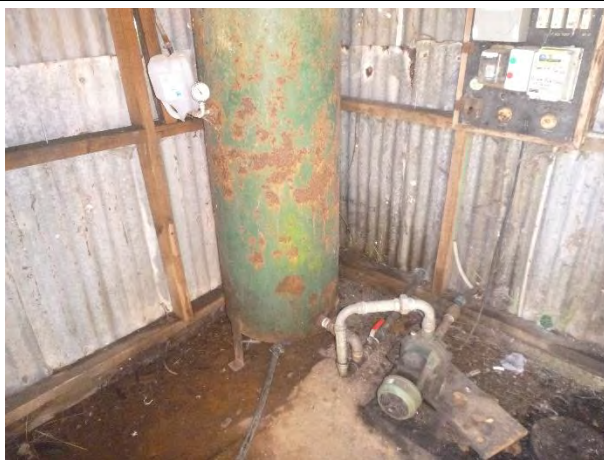
Photo 33: Inside metal shed.
