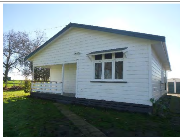
Photo 4: Western side of the residential dwelling.
