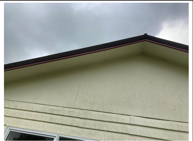
Photo 34: PACM – gable end cladding on dwelling
