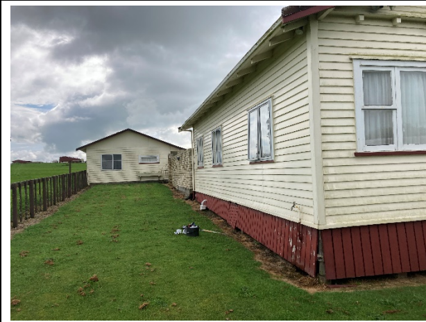
Photo 35: Residential dwelling located in south-western corner of the Site
