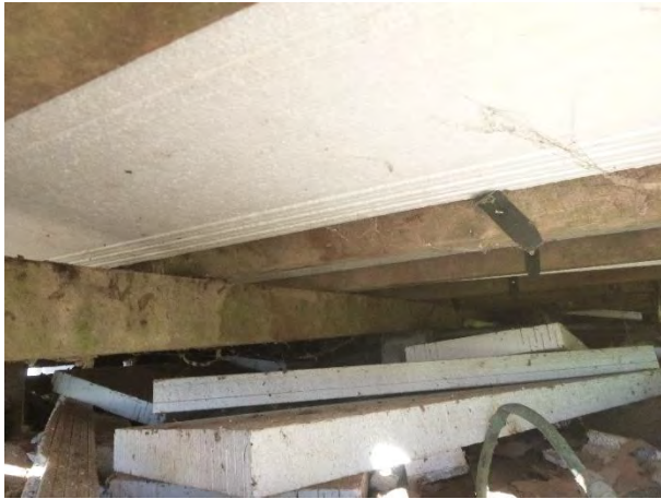
Photo 7: Insulation material beneath the dwelling.
