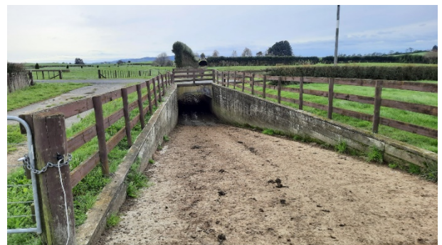
Photo 30: Tunnel for Cow traffic – Located North-Eastern Corner of the Site
