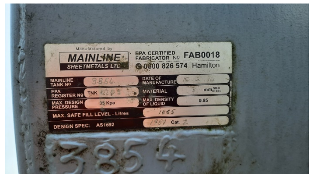
Photo 10: Label on Above Ground Diesel Tank
