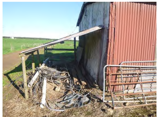
Photo 16: Extension off farm shed used to store timber, PVC pipes and farm fencing.
