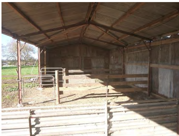
Photo 15: Inside metal farm shed.
