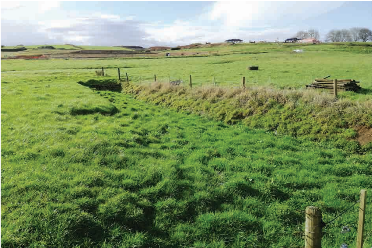
Figure 7. Example of erosion and land modification (access way).
