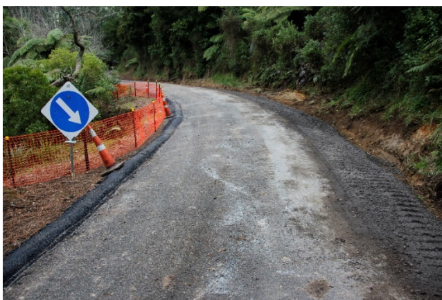
Figure 2 Temporary repairs showing safety fence, bund and widening
