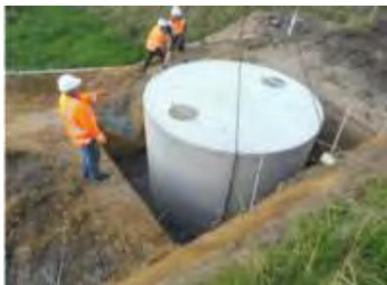
Photo 2: Tank in the hole
