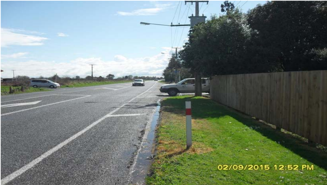
View of vehicle leaving entrance way and pole – facing north
