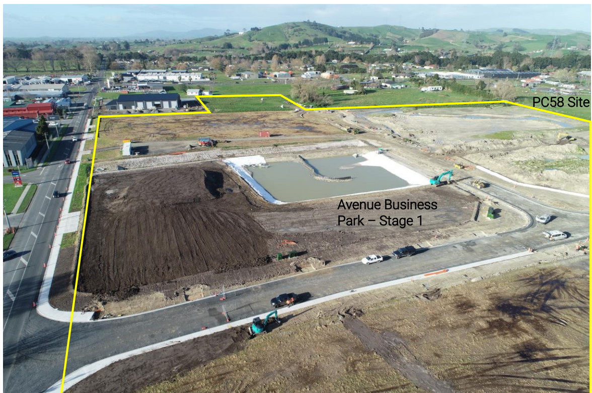
Figure 3: Avenue Business Park – Stage 1 (flown July 2023)
