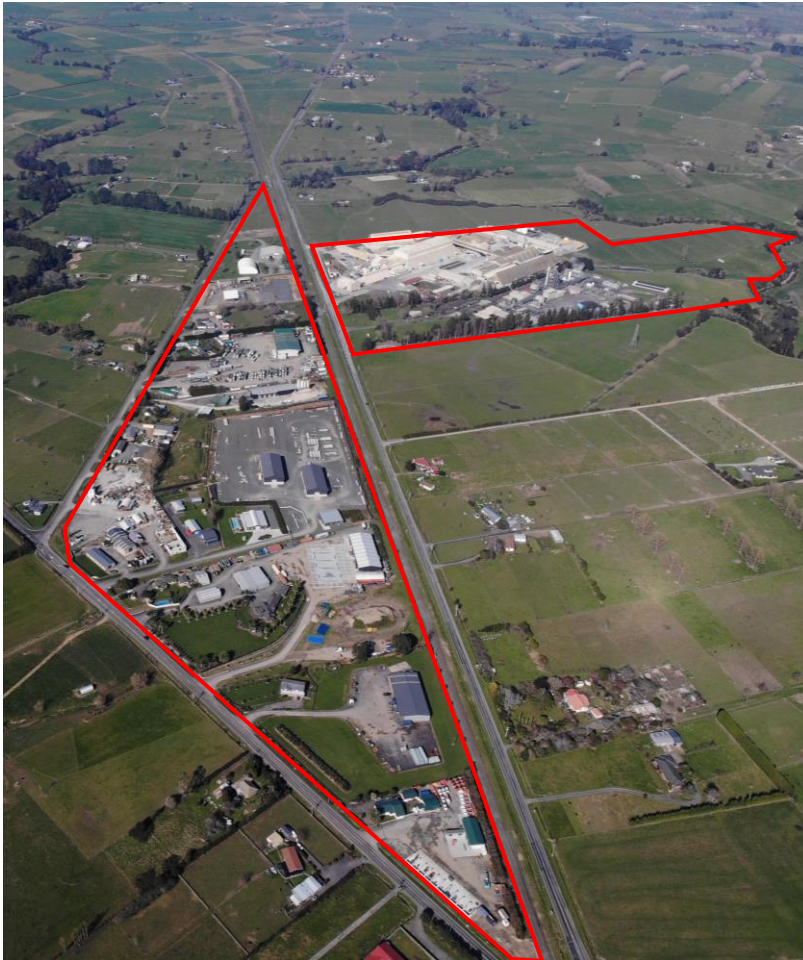
Figure 6: Morrinsville South industrial area (flown August 2023)
