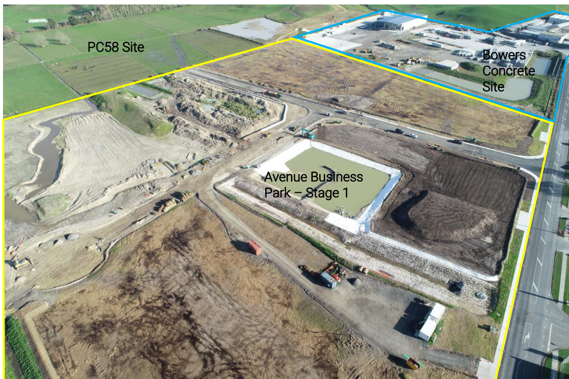
Figure 2: Bowers Concrete Site and Avenue Business Park – Stage 1 (flown July 2023)
