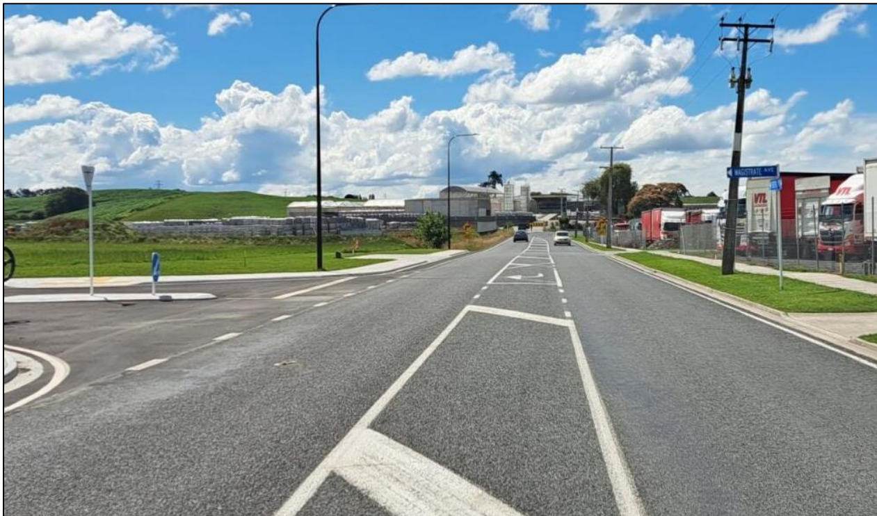
Figure 5 New intersection, showing flush median and space for right turning vehicles
