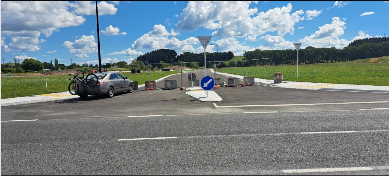
Figure 2 New intersection on Avenue Road north (photos from site visit 7 January 2024)
