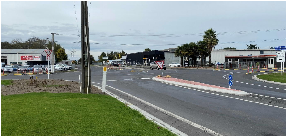
Figure 6: Avenue Road North approach to the SH26 roundabout
