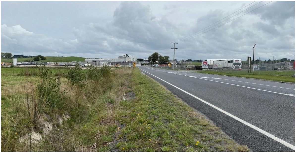
Figure 15: Sight distance from the new intersection to the north
