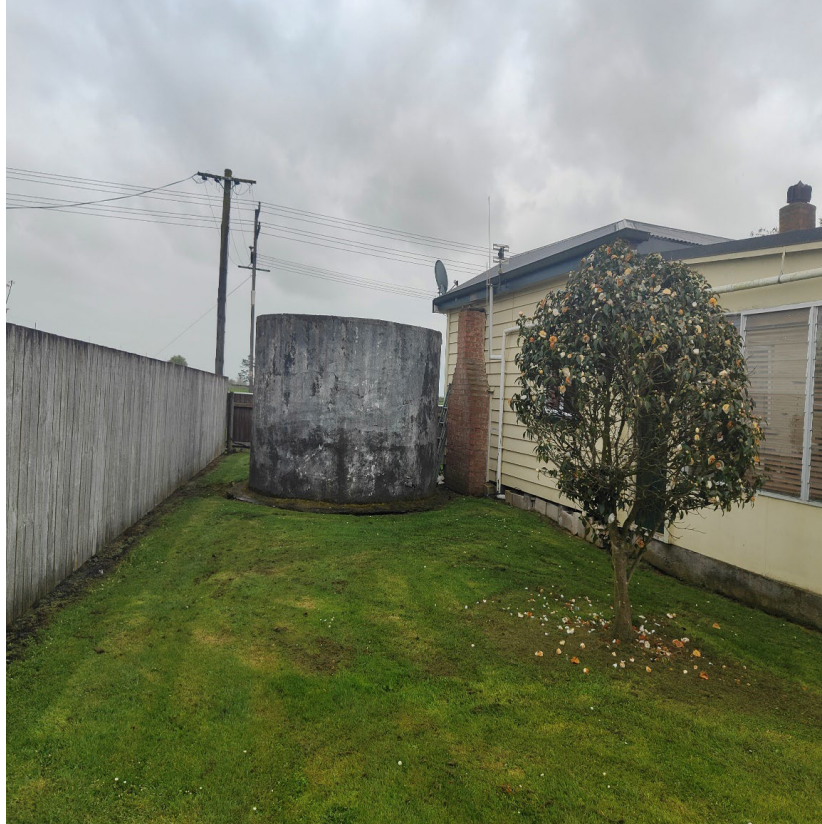
Figure 8 - 47 Farmer Road Tank Location
