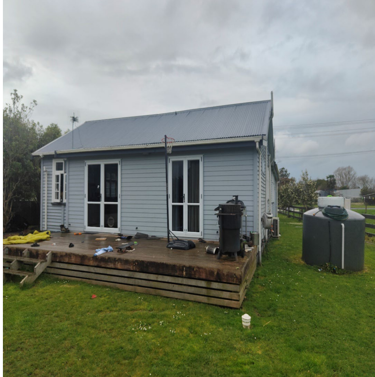
Figure 5 - 40 Farmer Road Tank Location
