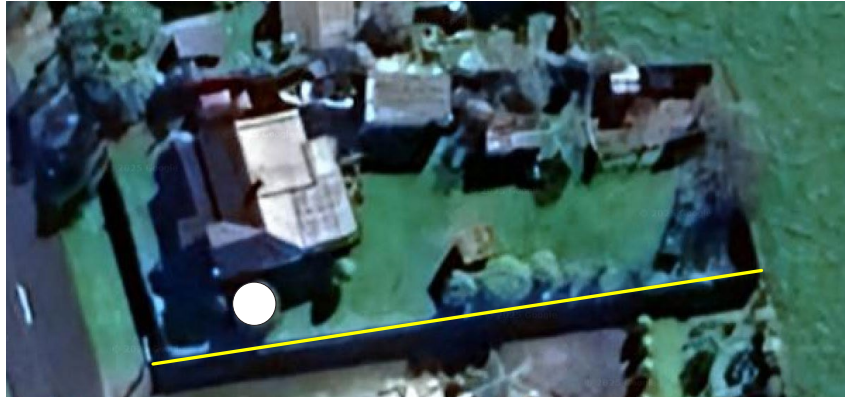
Figure 7 - 47 Farmer Road possible tank location
